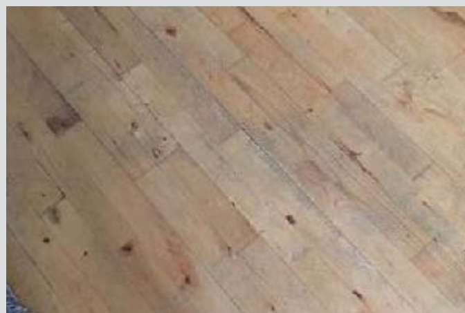
Worn floors: Photo from the surveyor's report, 2018. "The original floors are worn and creaky"
